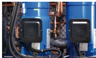
Scroll compressors (increased energy efficiency, reduced noise levels).
